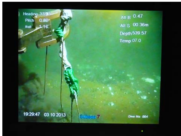
Installation with the ROV
