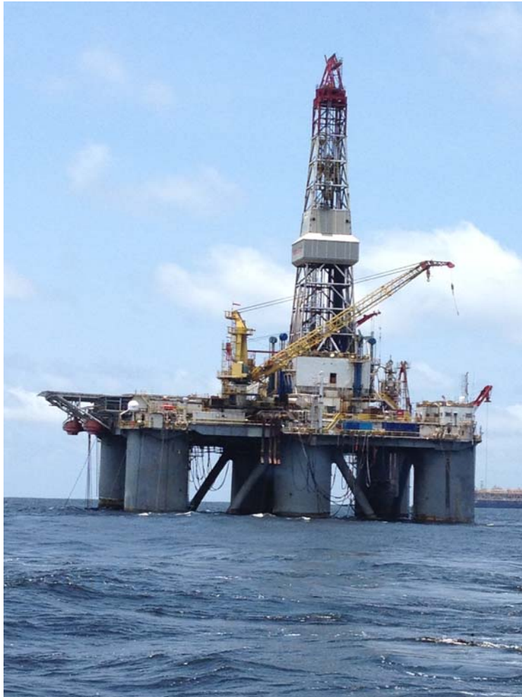
Drilling Rig GSF135
