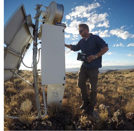
Installation PolaRx5, UNAVCO*
