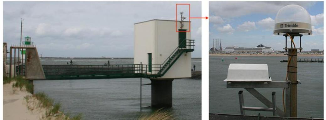
**Fig. 1** Example of a collocated transponder-GNSS installation at a tide-gauge in IJmuiden, the Netherlands
