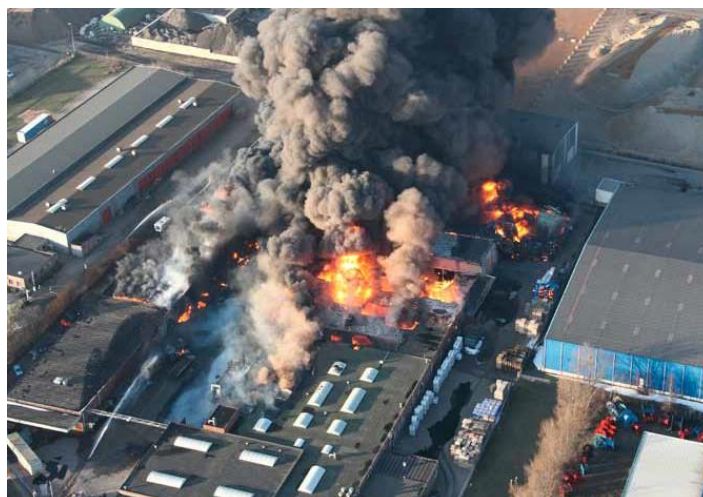
Figure 12 – The Fire on a chemical storage and packing plant Moerdijk.
